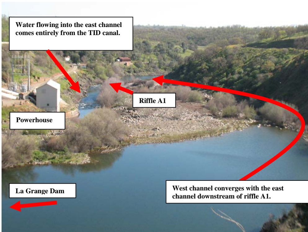
Figure 19. Downstream view taken during normal flows showing the junction of the east and west channels near riffle A1. March 12, 2009.
